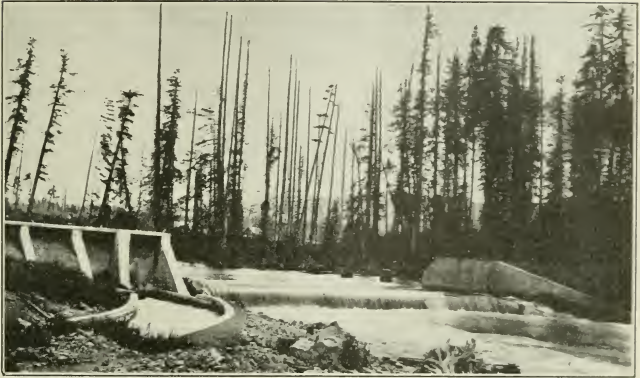
Diversion dam showing flume to intake, of Puntledge River Hydro-Electric Installation on Puntledge river about two miles below impounding dam.
